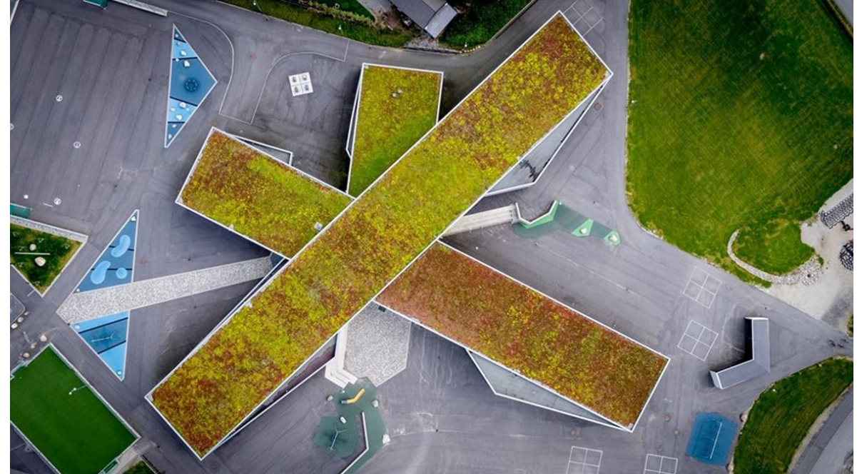
Green roof designed by Bergknapp – A Norwegian company producing green roofs and green walls
